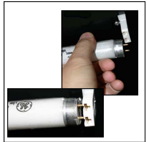
Above Photo Illustrations show removal of Fluorescent Bulb .
